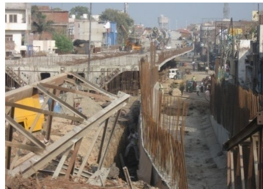
Fig no.83: Elevated road work under progress
