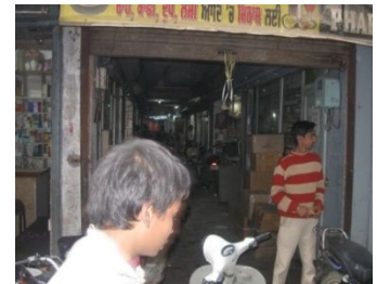
Fig no.52: Conversion of building into commercial shops
