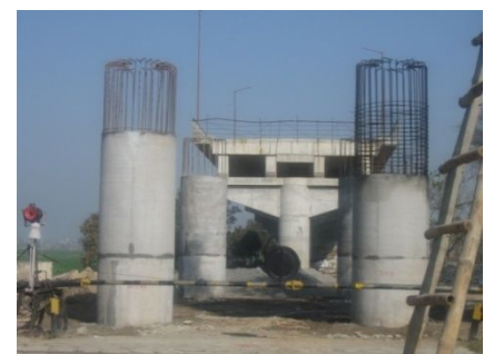
Fig no.81: ROB under construction
