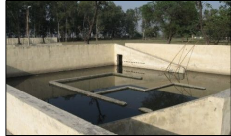
Fig no.89: Disposal Work, Fatehpur
