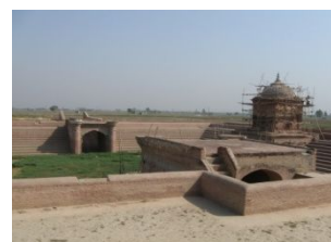
Fig no.50: Pul Kanjri under renovation
