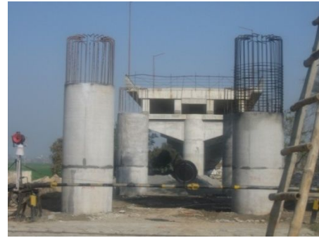
Fig no.84: ROB at Approach road to Baba Bakala Under progress
