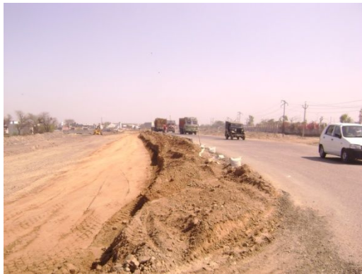
Fig no.82: Bye-pass work under progress
