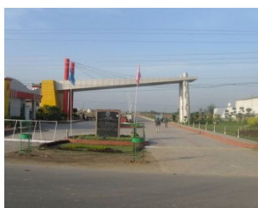
Fig no. 13 Upcoming mega project Shubham Enclave
